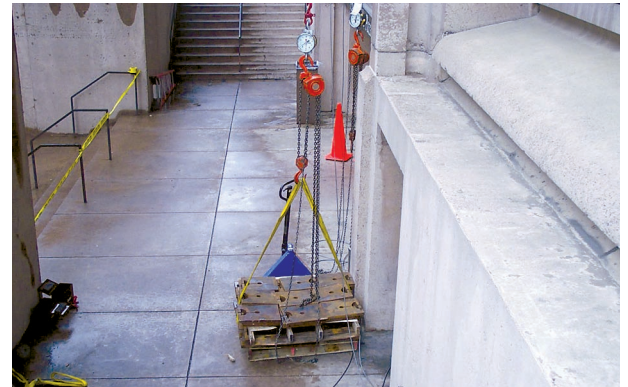
Suspended weight with dynamometer scale to load test davit arm
